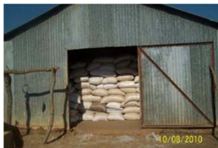
Chiyobola Community - Sibanje Shed, Monze District, Southern Province
